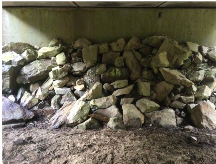
Right Bank Abutment when facing downstream
