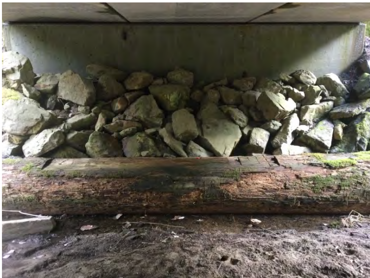
Left Bank Abutment when facing downstream
